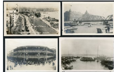
902 1920s eleven photos of Shanghai scenery, including The Sincere Company on Nanjing Road, Waibaidu Bridge, Bubbling Well Road (now West Nanjing Road), the Bund and Huangpu River, etc. Average size: 8.5x13.5cm
